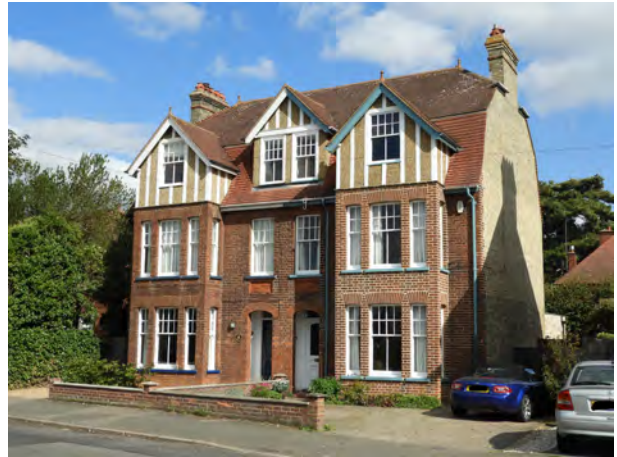
Victorian semi-detached villas, Needingworth Road, St Ives
