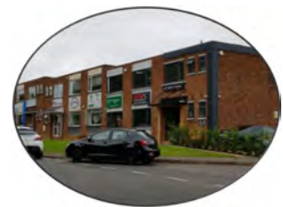
Mere View industrial units
