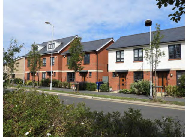
Diverse homes along Great High Ground overlook the open space associated with Fox Brook
