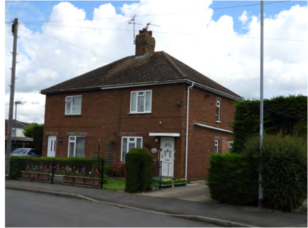
The post-war semi-detached homes create a very regular pattern of development along West Avenue
