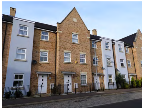
Three storey townhouses in Buttercup Avenue are designed to make efficient use of land
