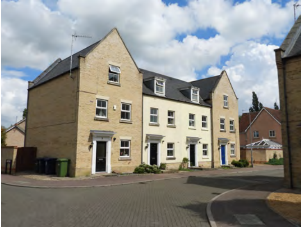
Signal Road 3 storey modern homes
