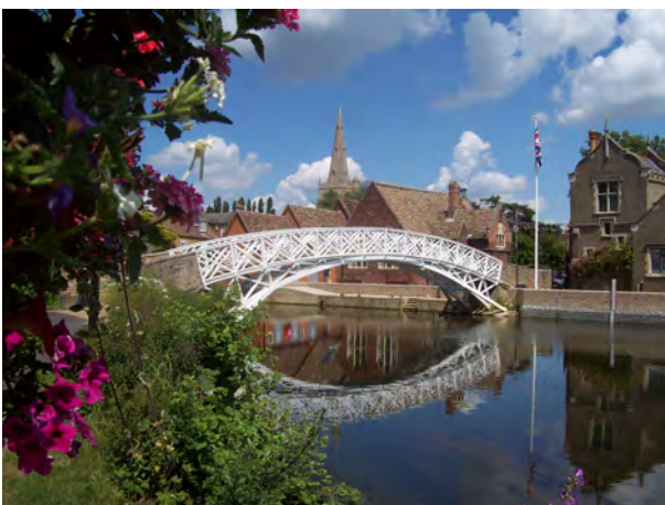
The Chinese Bridge provides access past Queen Elizabeth School and the Town Hall to the recreation ground
