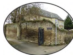
Priory barn walls
