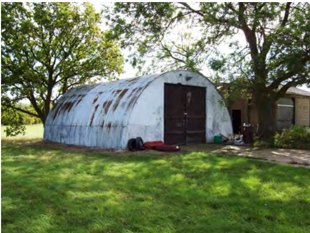
Little Staughton airfield nissan hut
