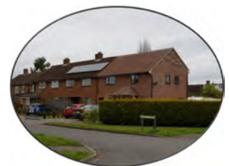
New build on Mandeville Road
