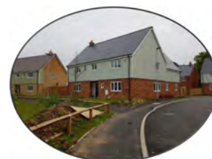
Park Close property with a distinctive mix of colours and materials
