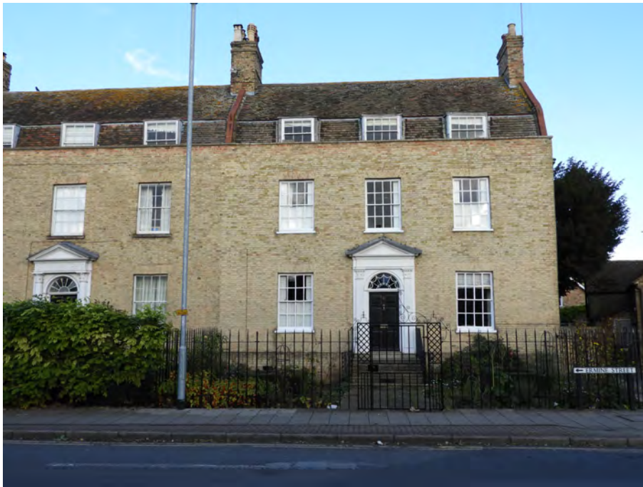
Late 18th Century gault brick town house at 79 Ermine Street, Huntingdon
