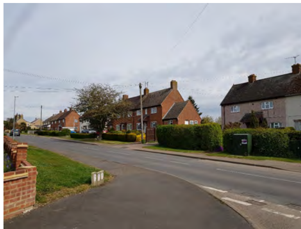
Early to mid 20th century housing, typically semi-detached with generous front gardens are found along Green End Road
