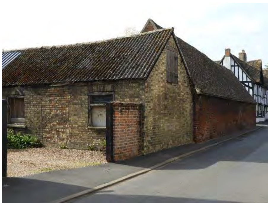
Gault and red brick barns adjoining a timber framed farmhouse, The Gables, Godmanchester
