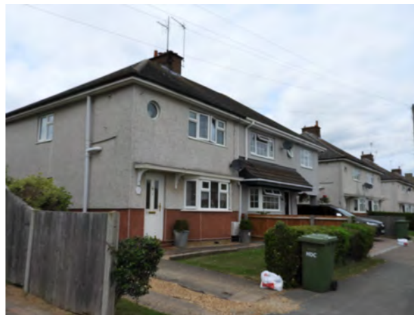
Station Road interwar semi-detached properties
