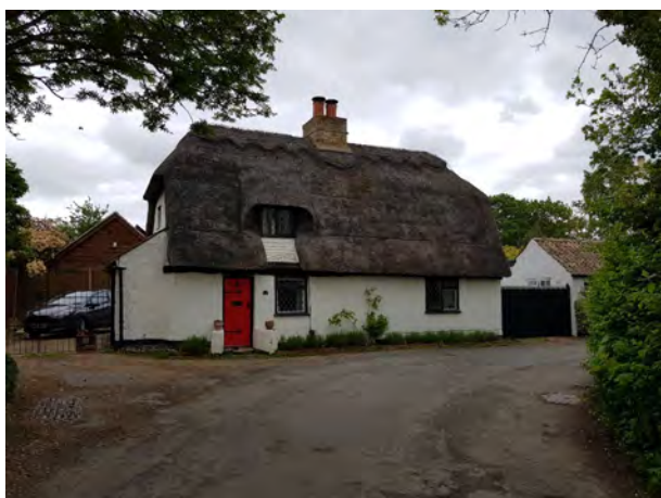
There are several cottages found within Fenstanton, some have thatched roofs
