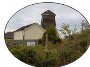
Mill Cottage and the Old Mill
