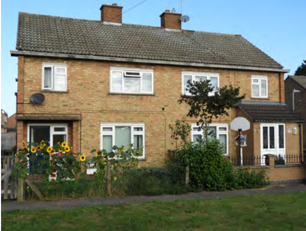
Semi-detached houses are the most frequently found form in this area with most pairs separated by driveways or garages
