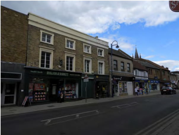
The High Street contains a wide variety of buildings and strong historic characteristics above the ground floor shop frontages
