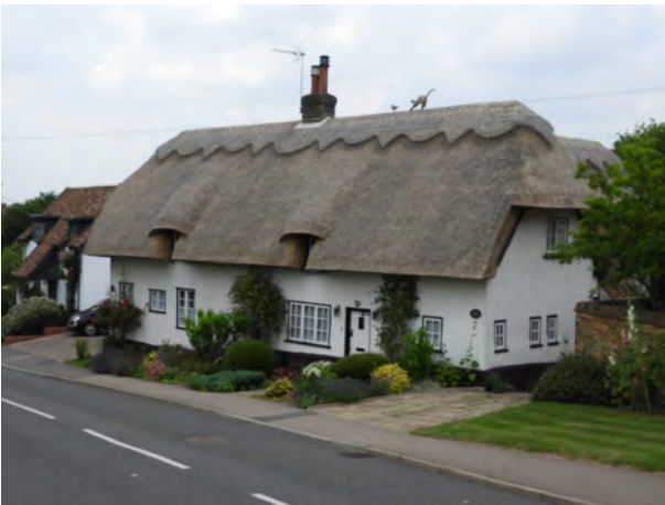
Homes in village centres are often traditional vernacular as found in High Street Abbotsley
