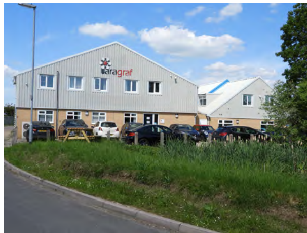
Unit within the West Newlands Industrial Estate constructed from a mixture of buff brick and cladding
