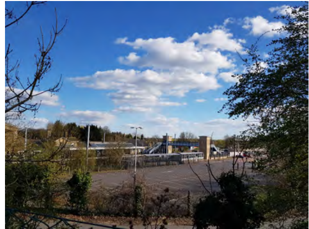
Huntingdon train station
