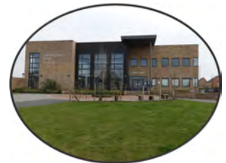
Godmanchester Bridge Academy
