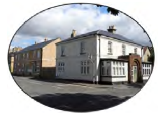
The former PH and modern infill behind in West Street
