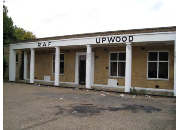
RAF Upwood contains a wide range of former military buildings, mostly of utilitarian architecture, vandalism and decay are damaging the historic character of the site
