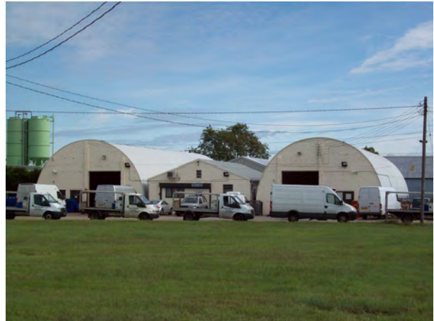
Some original military buildings remain at Little Staughton Airfield but most is now used as a solar farm
