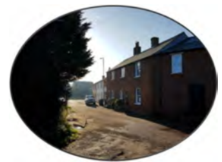
Terraces along Hardwick Lane with A1 access
