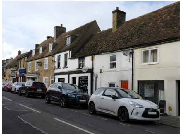
Great Whyte contains an attractive mix of building types with pastel render being a strong feature interspersed amongst buff brick
