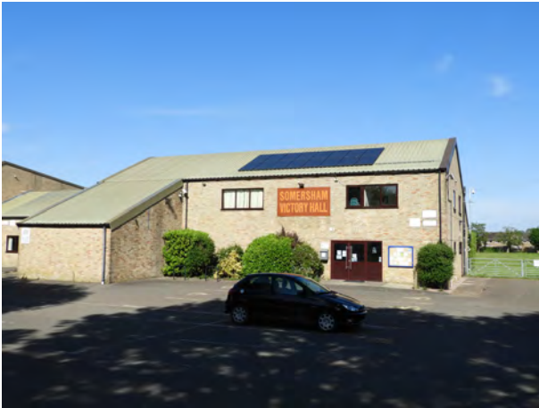
Somersham Victory Hall
