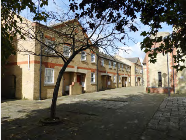
Modern infill development can blend sympathetically within a historic environment as achieved in homes adjoining Paines Mill
