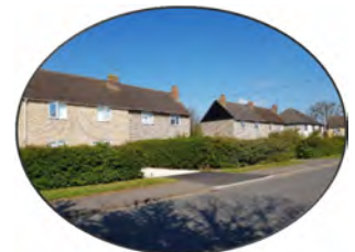
Silver Street with modern additions
