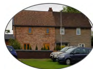
Property where concrete panels have been replaced
