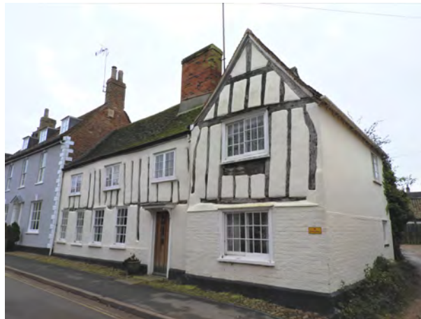
East Street includes a mixture of timber framed and Georgian fronted properties with some retaining shop windows and archways indicating historic commercial uses
