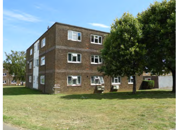
Low rise flats off Duke's Road are set in extensive open space with footpaths linking throughout the local area
