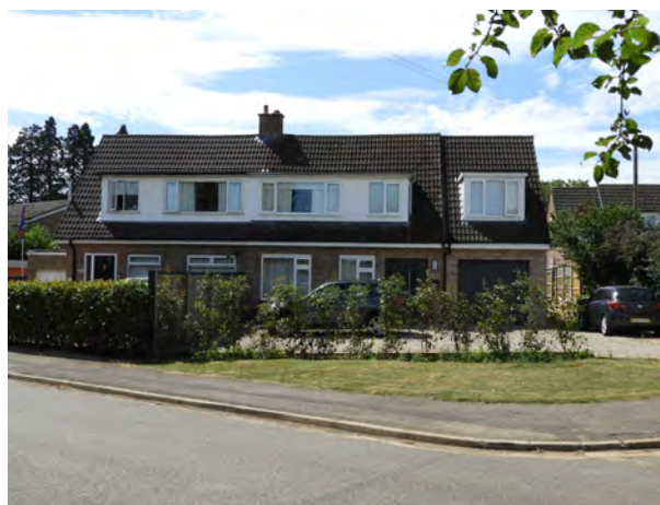
Side extension on a semi-detached chalet style home in Wilkinson Close
