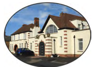
Converted Police Station on Blenheim Road
