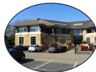
Offices at Parsons Green
