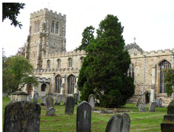
St Mary's church, Eaton Socon is largely 15th century in appearance although much was rebuilt in the 20th century after fire damage, the four stage square tower forms a strong feature in local views
