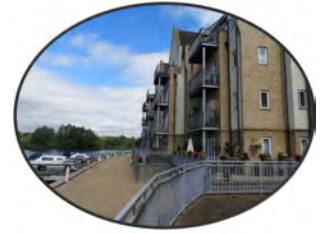
Apartments by moorings
